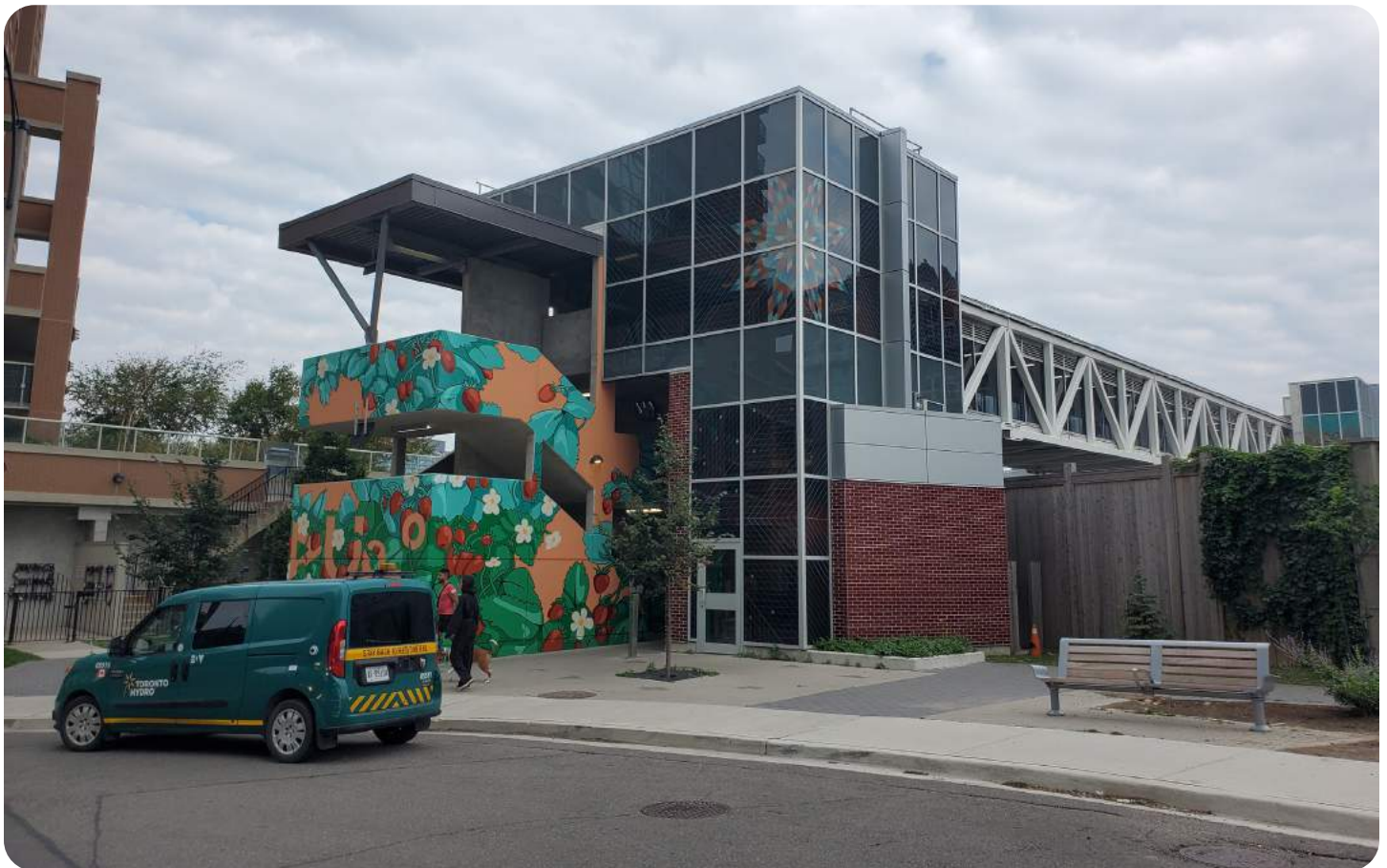
Pedestrian Bridge looking northwest
