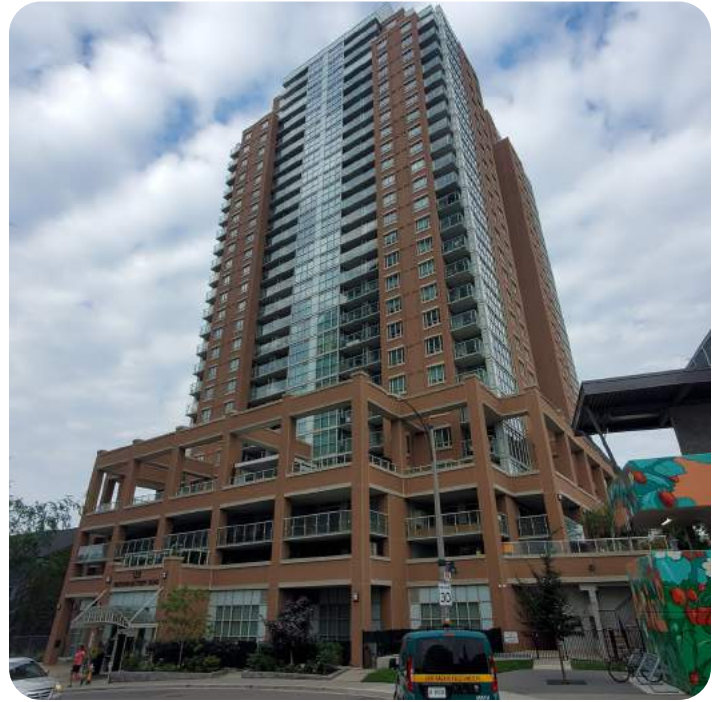
125 Western Battery Road looking west
