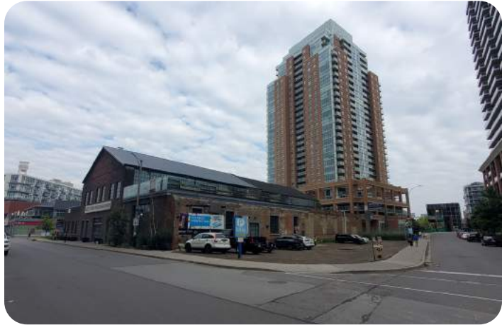
Subject Site looking northwest from Lynn Williams Street
