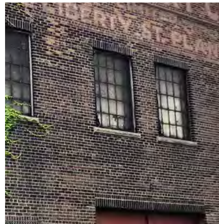
Figure 82. Original metal, single-glazed windows (ERA, 2023).
