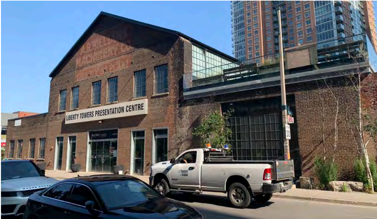
Figure 8. South elevation (ERA, 2023).
