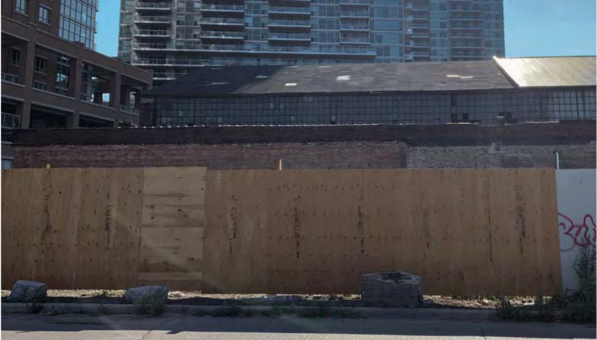
Figure 19. Northern portion of west elevation (ERA, 2023).
