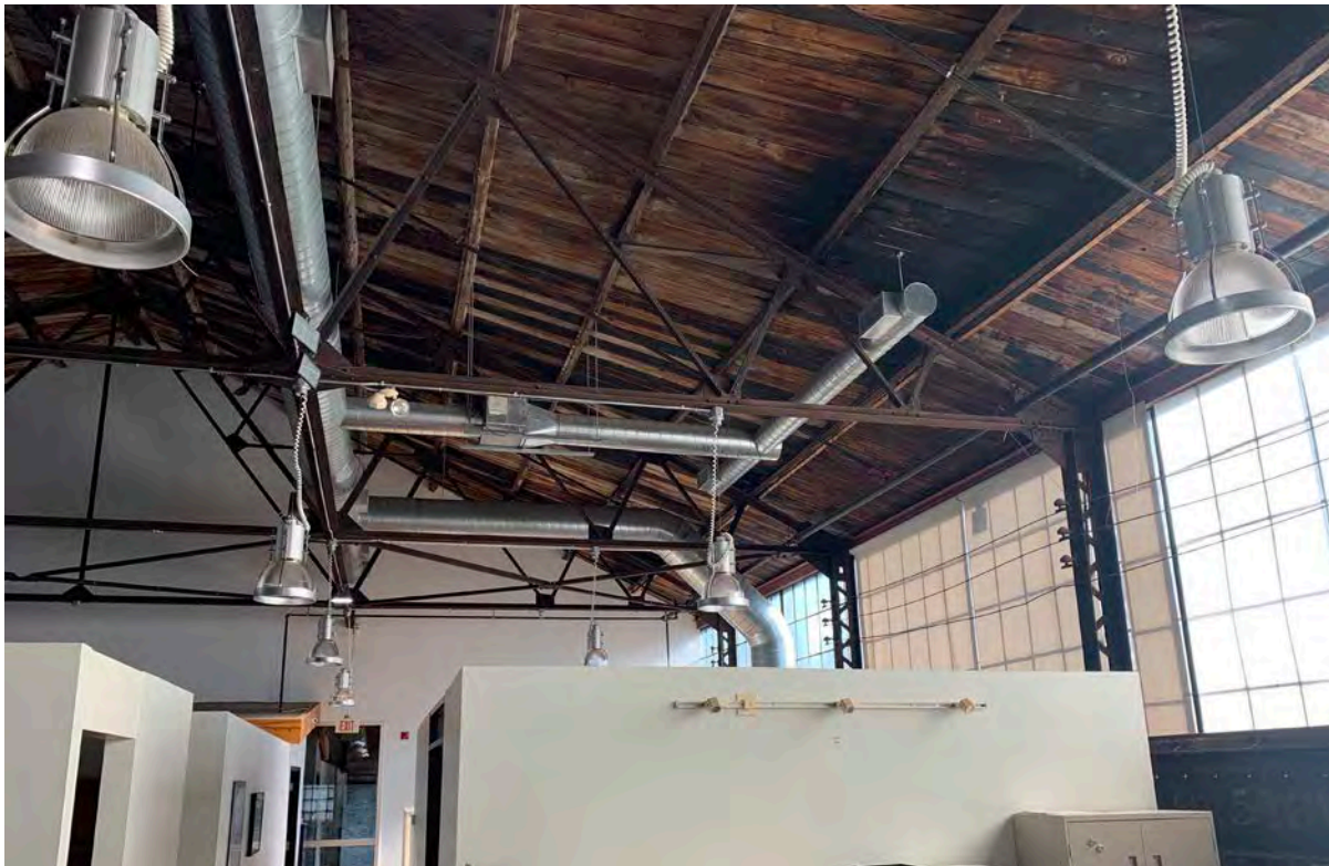
Figure 22. Interior of the second storey with the interior partition between the north and south portions of the building. The steel frame support and open span roof is visible (ERA, 2023).
