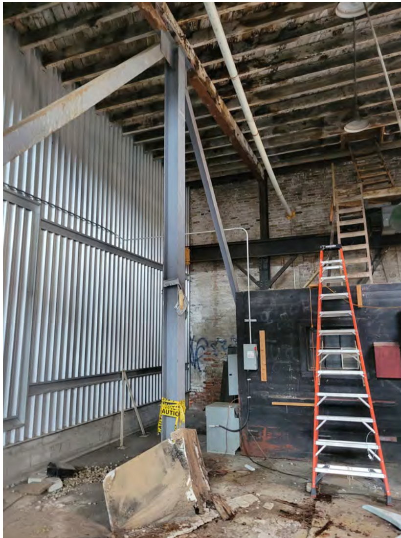
Photo 6: Existing vertical bracing installed in 2005 along grid line 7
