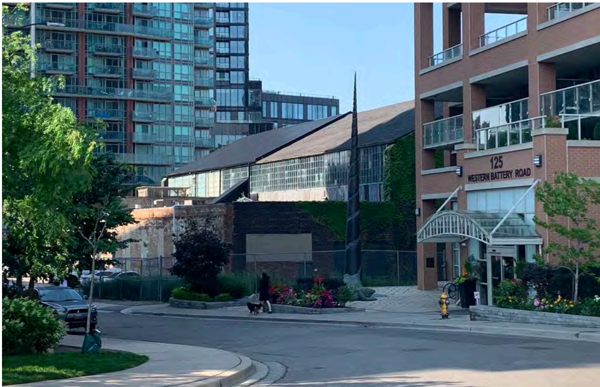
Figure 16. Context photo looking southwest along Western Battery Road (ERA, 2023).
