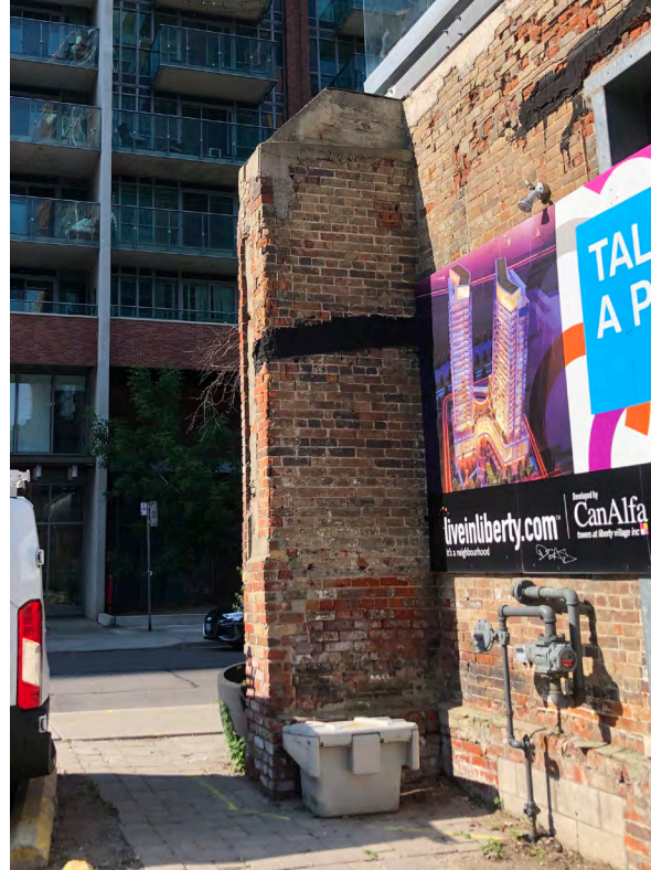
Figure 11. North elevation of wall remnant (ERA, 2023).
