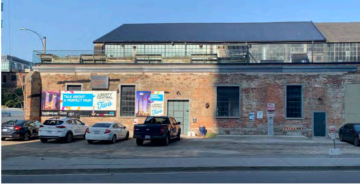
Figure 13. Southern portion of east elevation (ERA, 2023).
