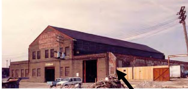
former Central Prison Paint Shop wall visible on right
