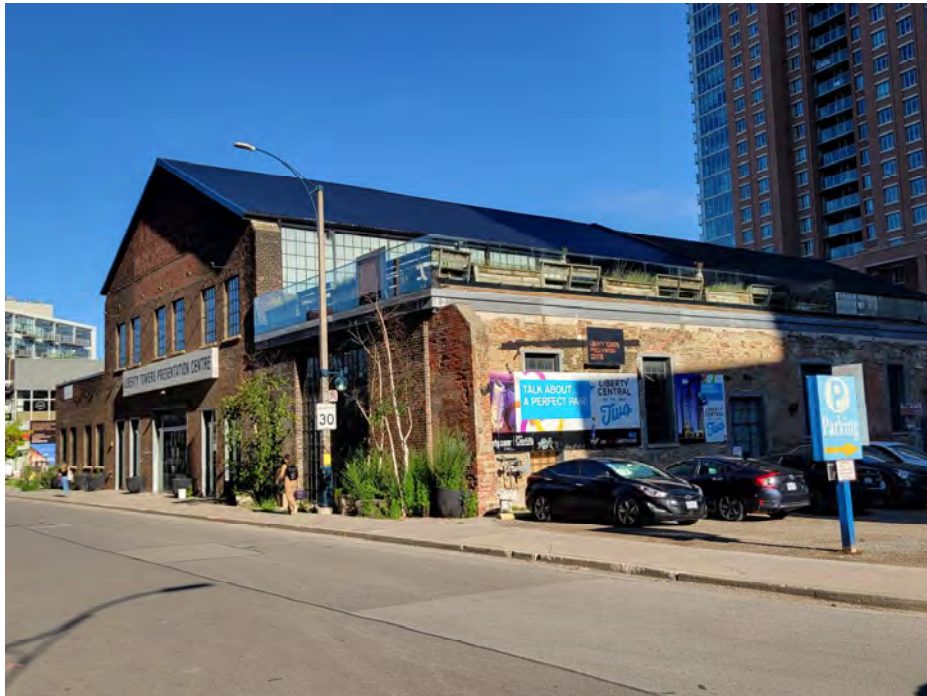
Photo 3: Overall view looking northwest
