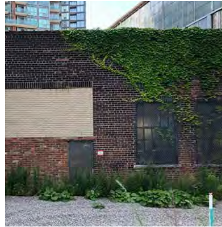
Figure 81. Detail of brown facing brick (ERA, 2023).
