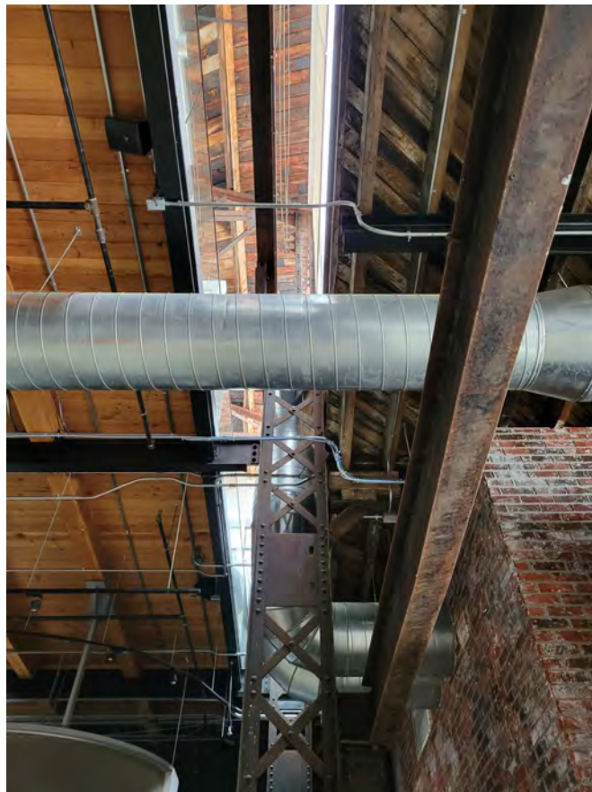
Photo 5: View of typical interior column
