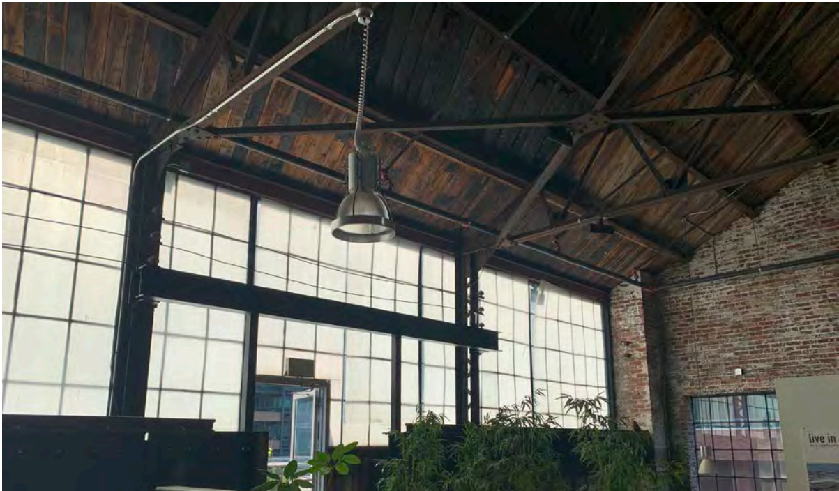
Figure 24. Interior looking southeast showing the clerestory windows on the southern portion of the building (ERA, 2023).
