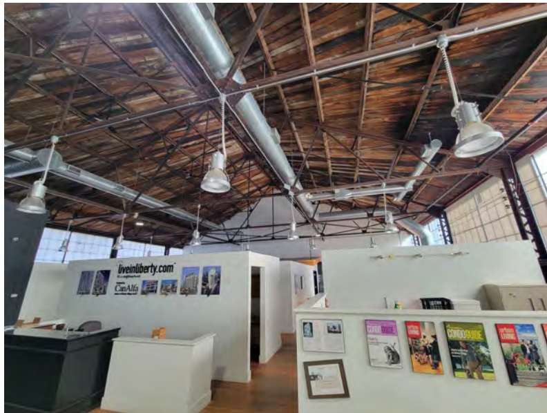
Photo 4: View of the interior at mezzanine level looking north
