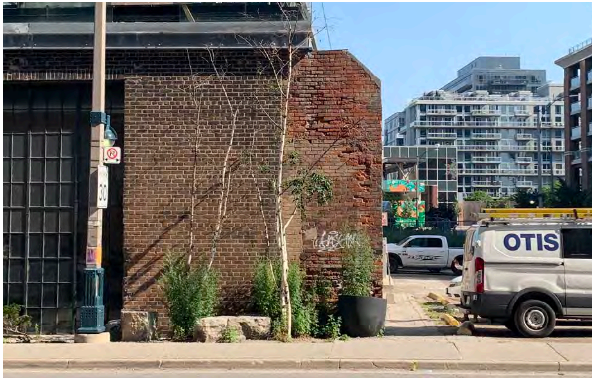
Figure 9. South elevation showing wall remnant (ERA, 2023).
