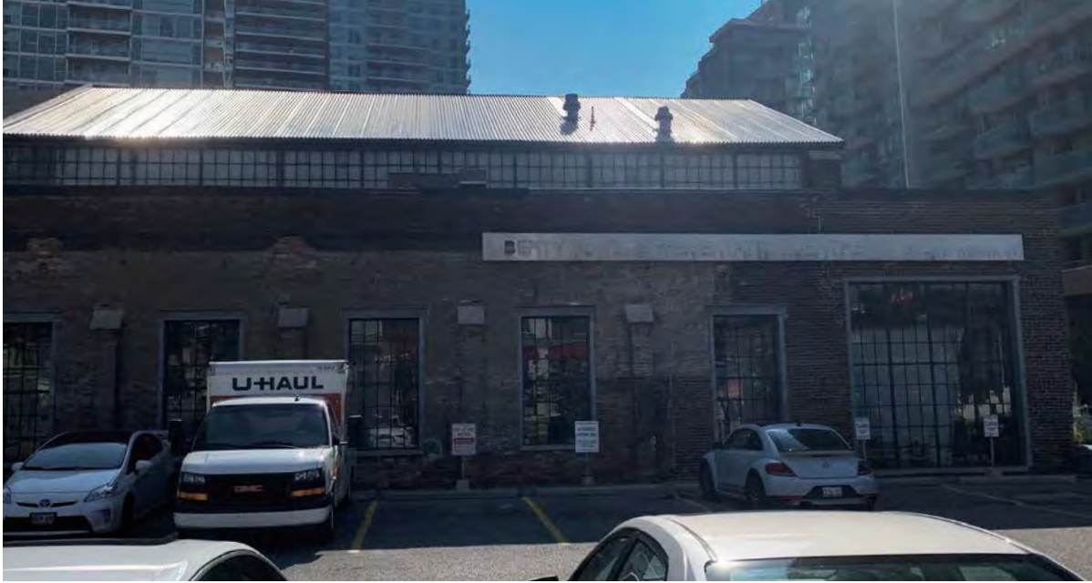
Figure 21. Southern portion of west elevation (ERA, 2023).
