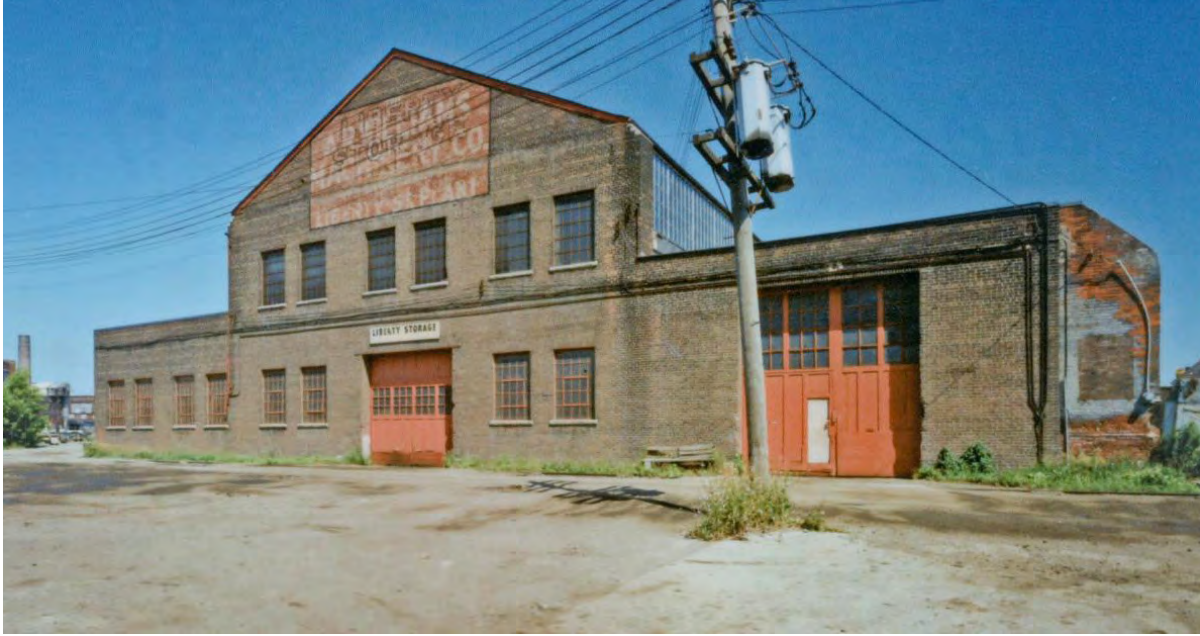
Figure 48. 1987 photo of the south elevation of the Site. The remaining portion of the Broom Factory/Paint Shop wall is visible to the east (right). The large opening on the eastern portion of the south elevation may have been used for a railway siding (Toronto Public Library).
