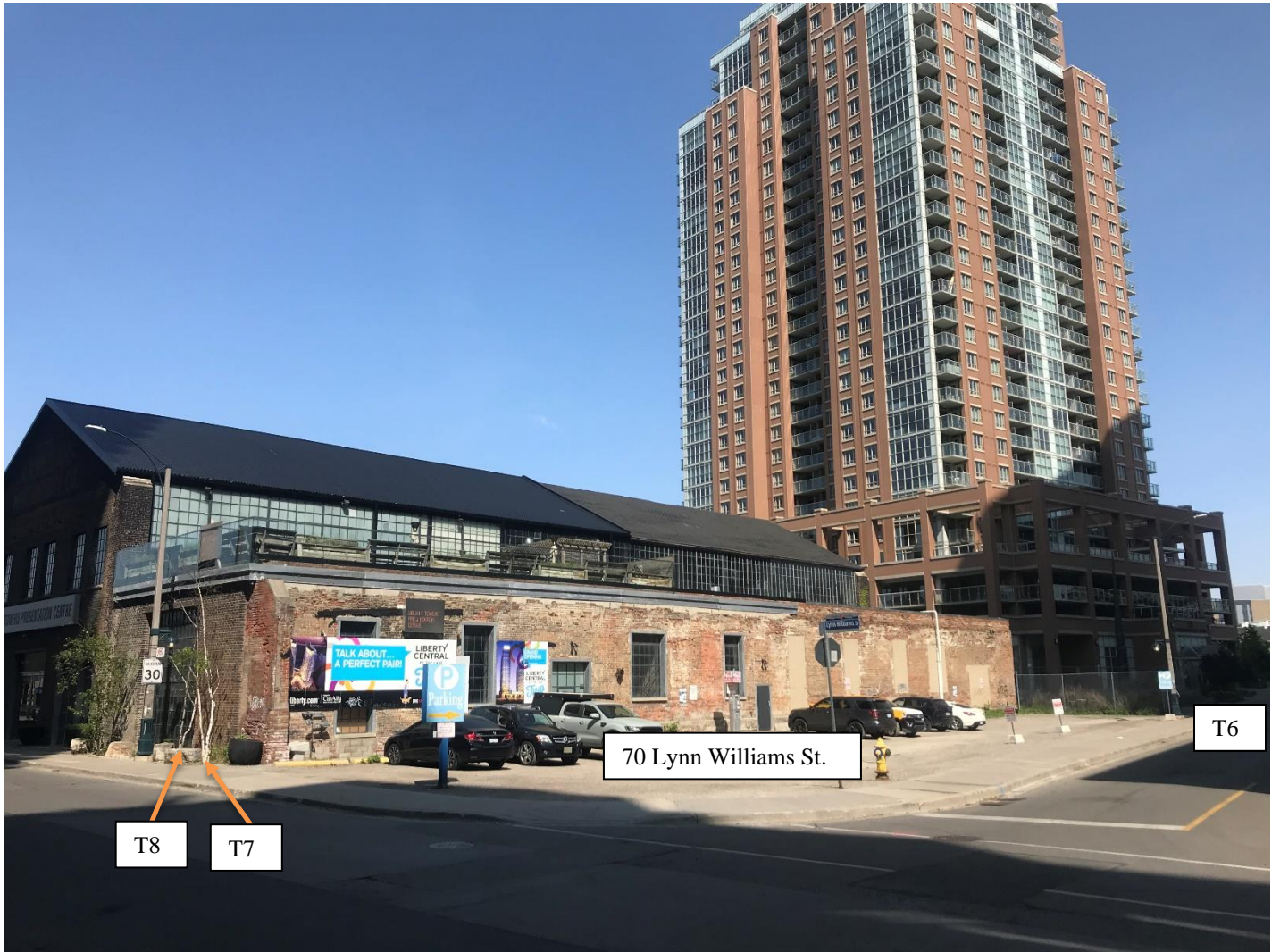
Photo 7: 70 Lynn Williams St. (facing northwest)
